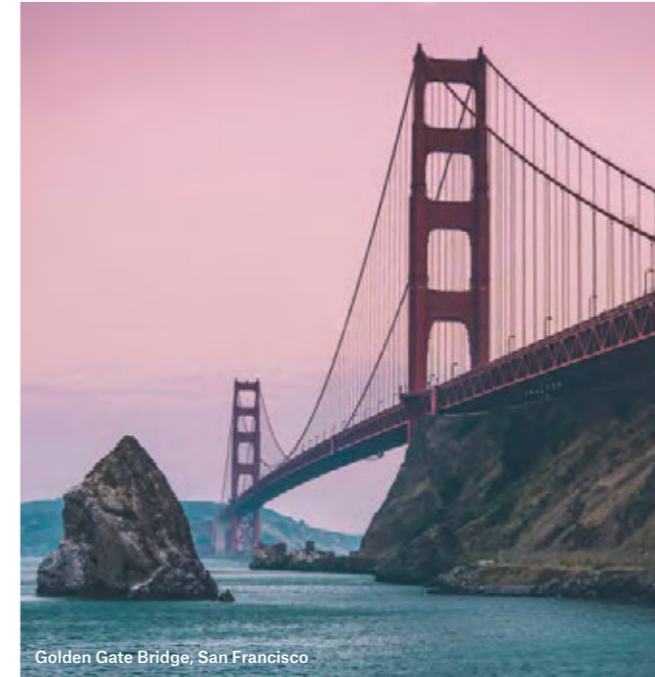
Golden Gate Bridge, San Francisco
